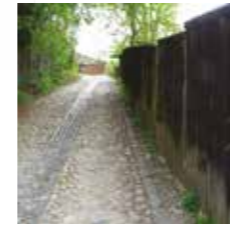
Good quality pavement
