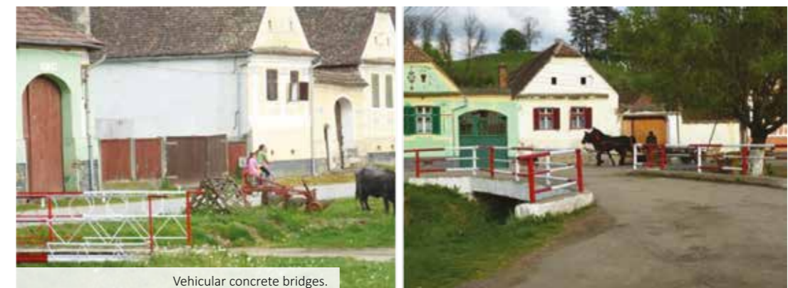
Vehicular concrete bridges.
